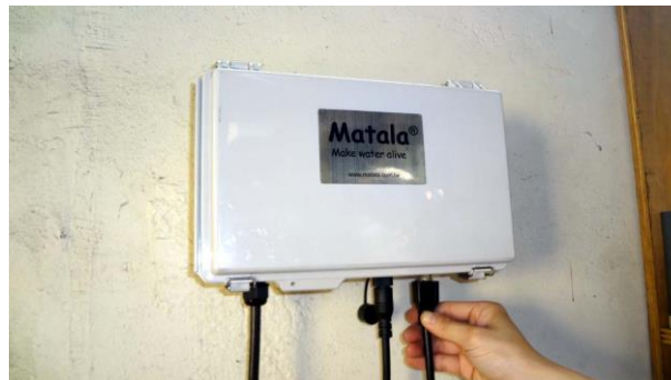
8, Connecting the pump power cord
