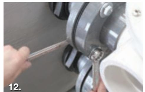
en to 20-30 ft/lbs. The flanges will not contact each other as the gasket between the flanges creates the water tight seal. DO NOT over tighten flanges.
