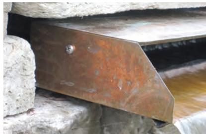
Figure 4 - Screw Placement
